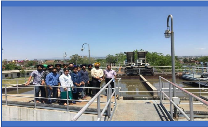
Industrial Visit to 30 MDL Sewerage Treatment Plant Organised by Mechanical Eng. Dept.
